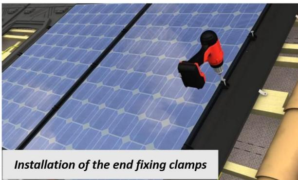
*Installation of the end fixing clamps*
