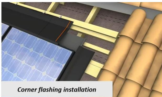
*Corner flashing installation*
